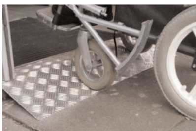
Temporary ramped entrance
